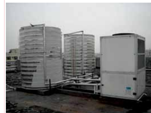
Air Source Heat Pump and Water Storage Tank
