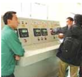
Fully Automatic Standby Power Management System Control Panel
