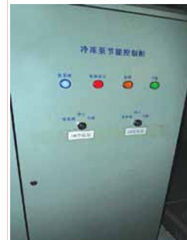
Control Panel of Chilled Water Pumps
